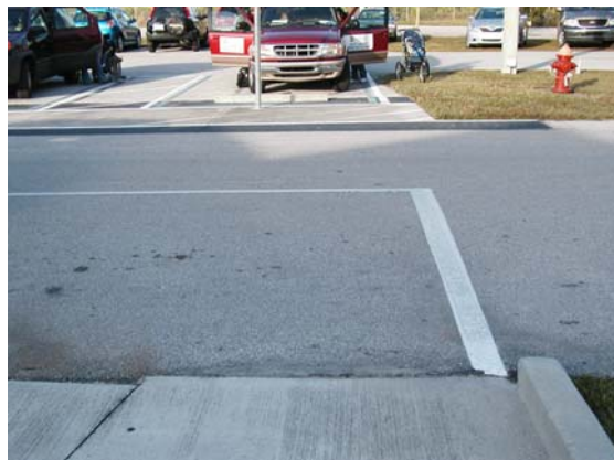
The existing curb ramp is not directly connected to handicapped parking spaces
